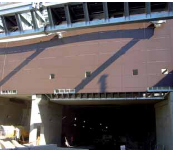
Tunnel NSBP Brisbane
