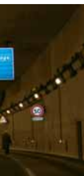
Tunnel Nanterre Paris
